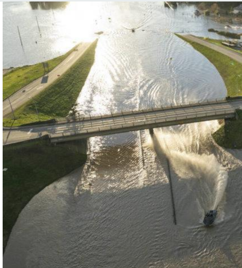
A boat speeds along a flooded highway 1 in Abbotsford, B.C., Tuesday, Nov. 16, 2021. THE CANADIAN PRESS/Jonathan Hayward
